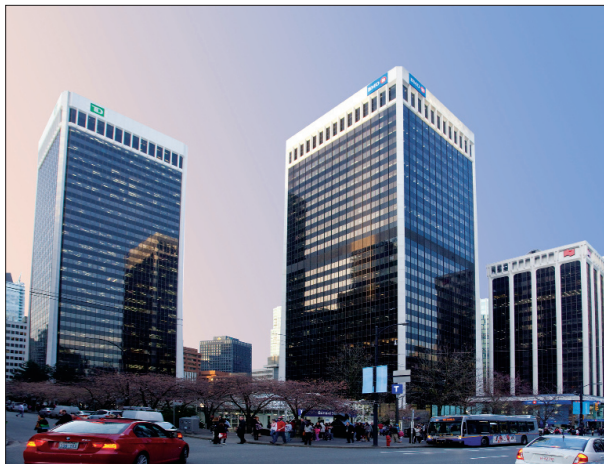
Bentall Centre demonstrates responsible property investing standards in its green construction and Go Green Tenant Action Committee
